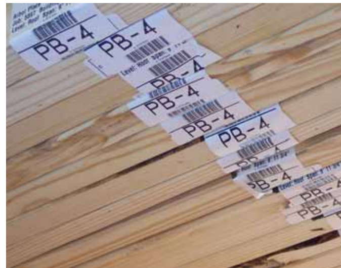
Individual trusses are tagged with details of their placement to help framers during installation.
