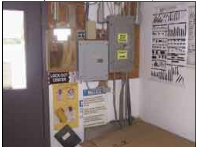
Lock out/Tag out device, safety policy and procedures manual and other warning signs in a typical shop settings.
