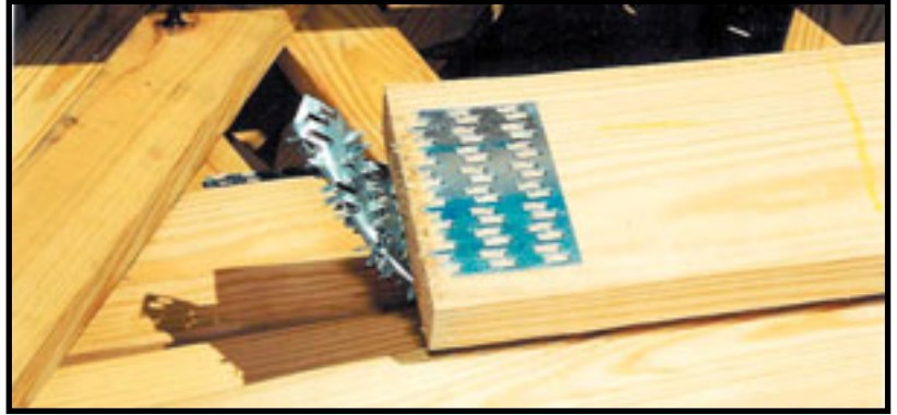
BROKEN BC SPLICE PLATE
