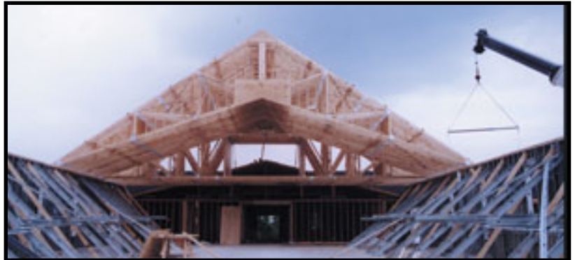
60' SCISSOR TRUSSES WITH PLYWOOD SPLICE AND BRACED WALLS
