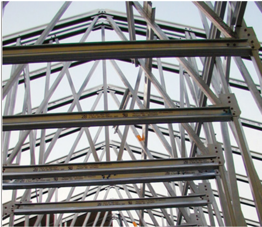
Notice the hall height built into the trusses and that lateral and diagonal bracing of the web members, which was also used as temporary erection bracing. Also, notice the STCA orange tags on the web members and the green tag as the bottom noting a bearing location.
