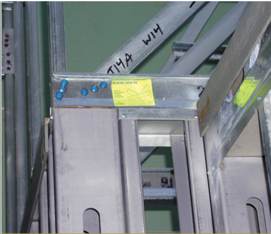
An STCA bearing location tag installation aid.
