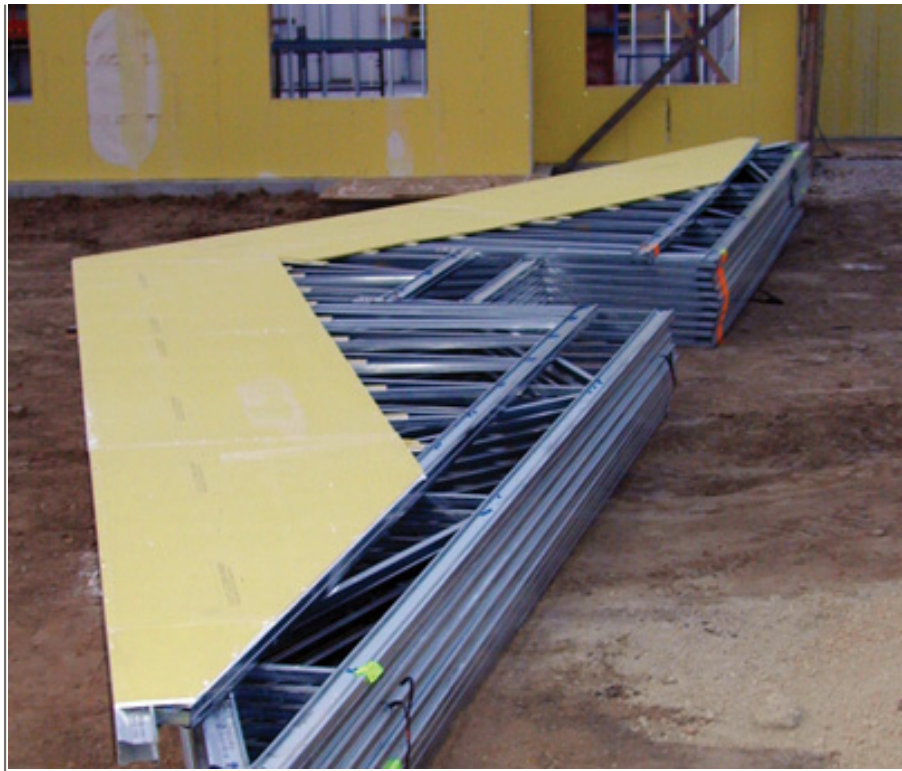
A pre-installed gypsum draft/fire stop.
