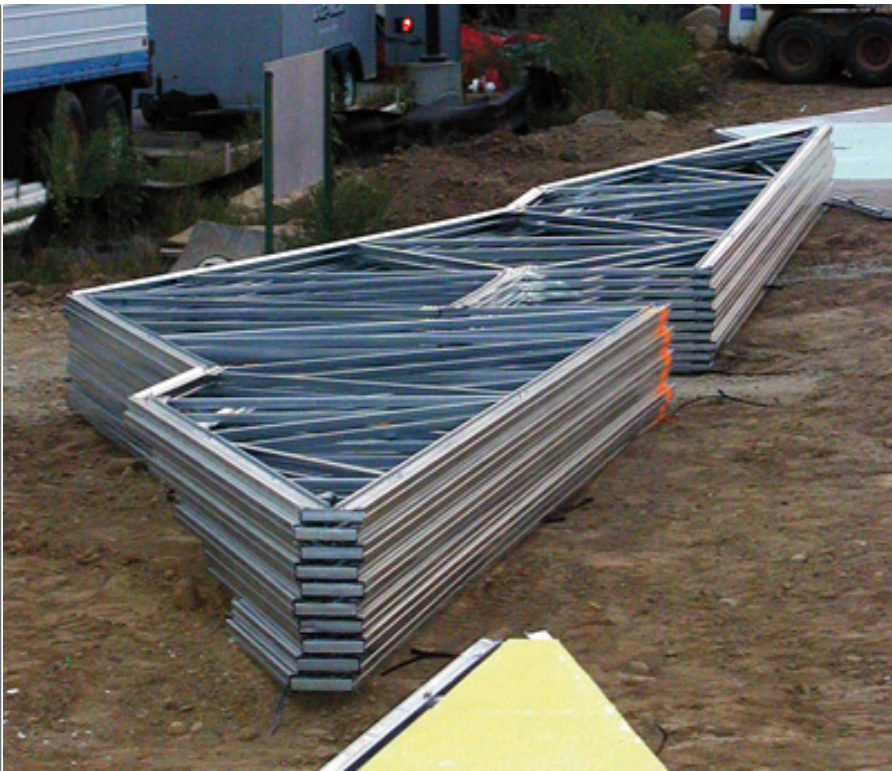
Note the top and bottom chord pitch breaks to meet the varying roof and ceiling profiles needed for the architectural appearance.
