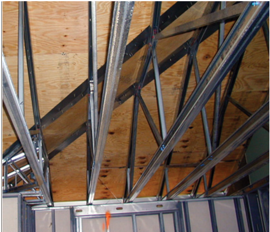
An interior view of the wall pop-out and roof valley condition.
