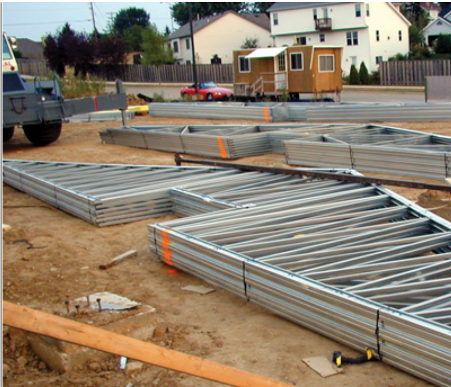
Trusses ready for installation using a spreader bar. Note the orange paint designating a bearing location.
