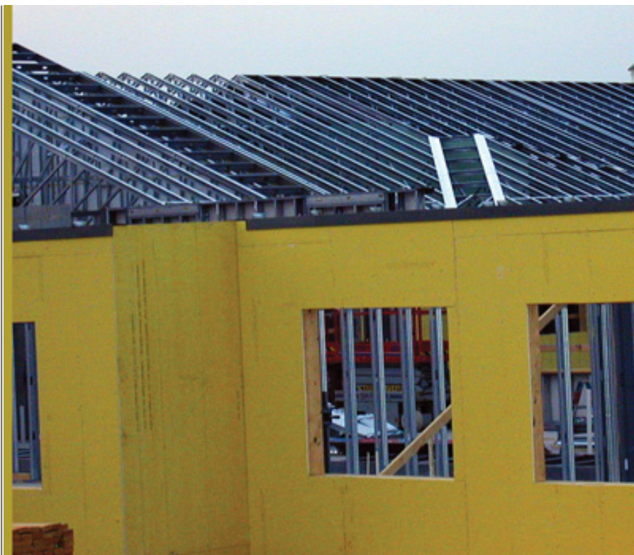
An exterior view of the valley condition unsheathed.
