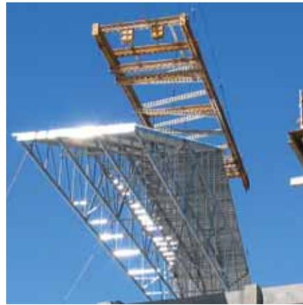
A section of pre-sheathed light gauge steel roof trusses are hoisted into place at a commercial jobsite in Birmingham, AL.
