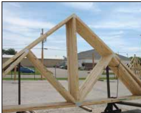
Vertical stacking requires sturdy back and bottom supports for storing the banded groups of trusses.
