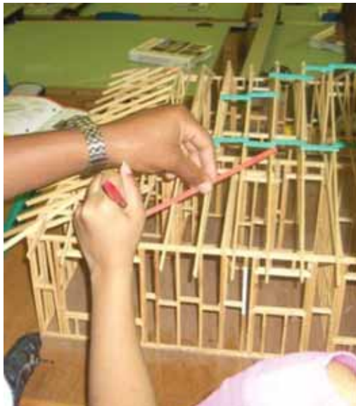
On one recent occasion, a class had the chance to apply temporary bracing. Every time the kids set a support, they referenced BCSI B1 and B2.
