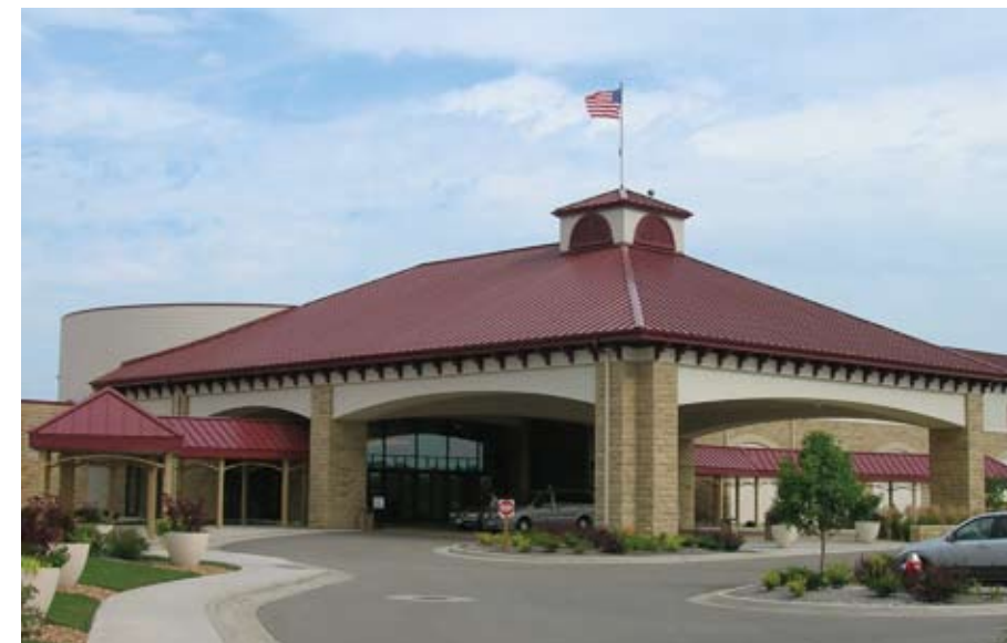
For this casino expansion project, converting cold-formed steel trusses was a "no-brainer."
