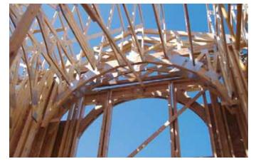
Nelson Truss, Inc. of Edgerton, WI supplied the roof trusses and I-joists for a 5000 sq. ft. custom home located west of Milwaukee. These intricate intersecting radius trusses resulted from the customer's desire for a dramatic ceiling design.
