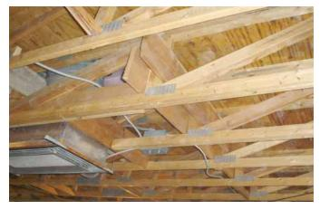
One WTCA member sent in these pictures of cut girder trusses discovered during the remodel of a local restaurant. A contractor who works regularly with this component manufacturer was doing interior remodeling and reroofing on the restaurant when they noticed a previous contractor had cut some of the girders. The contractor recognized the problem and immediately contacted the component manufacturer.
