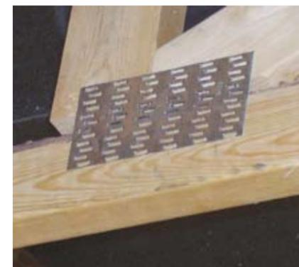
Figure 3. Wane under plate contact area of bottom chord.
