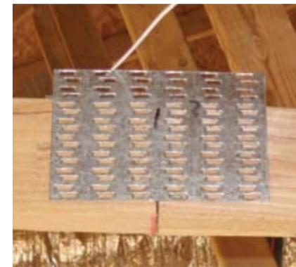
Figure 1. Plate misplacement. Engineering specified bottom edge of plate at the bottom edge of the chord.
