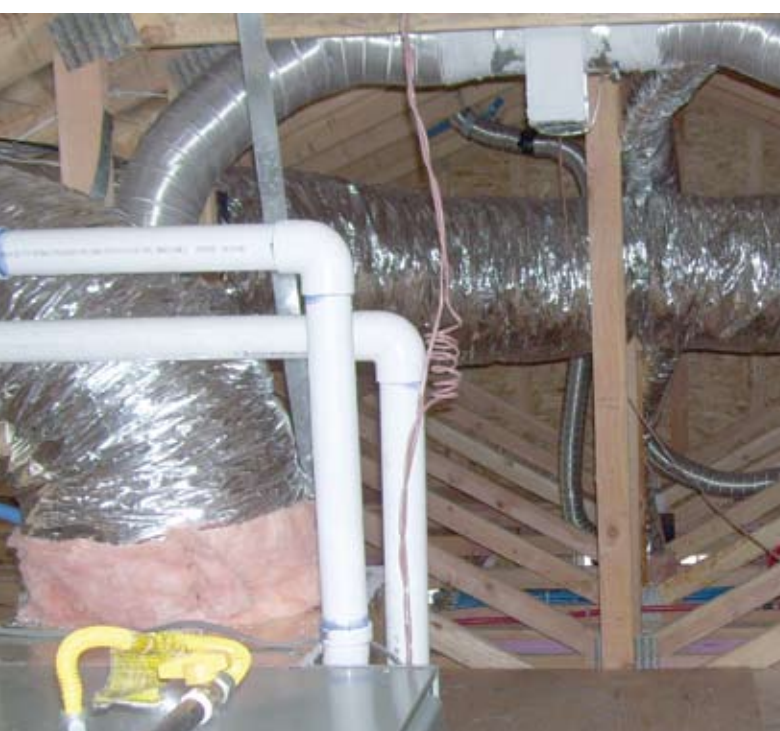
A tankless water heater is mounted to truss verticals. Utilizing this extra space in the attic meant the hot water lines could be limited to 20 feet or less.
