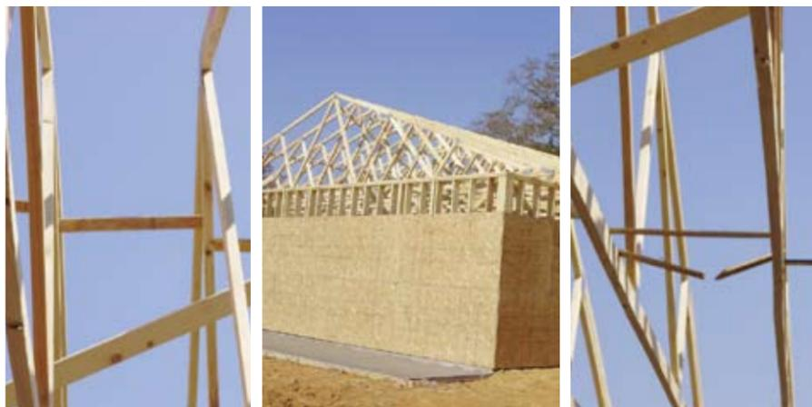
While traveling through southern Georgia, Glenn Traylor (ITW Building Components Group) ran across this project. The entire building is braced with ripped 1/2" x 2" x 24" OSB. "If the typical 2 x 4 or 1 x 4 braces are 'killer cleats' then this needs a new description," he said.
