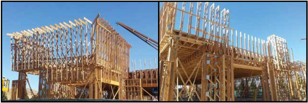
Photo 1. The builder completed this 5,000 square foot commercial mall project 30 days earlier than planned and saved $80,000.
