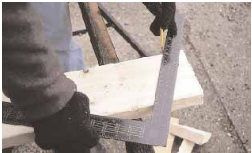
Figure 4. To make a double-cheek cut on a hip, the author lays out a plumb cut with a framing square. He marks both sides of the 1½-inch tongue on the square (above). Leaving the line visible on the board, he then cuts along the outside line with the saw set at a 45-degree bevel, moving from the top edge of the rafter towards the bottom to cut the long point (middle). Finally, he cuts in the opposite direction to cut the short point, resulting in a near-perfect double cheek cut (left).
