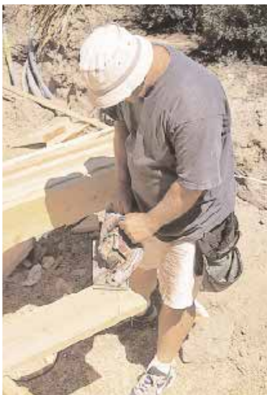
Figure 8. The author cuts the jacks for all four hips in a roof in sets (four hips require eight jacks of each length). The photo above shows the setup for the longest jacks. Similar setups would be required for each of the five jack lengths in the example roof.
