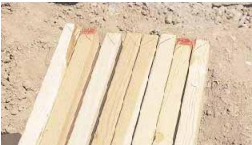
Figure 8. The author cuts the jacks for all four hips in a roof in sets (four hips require eight jacks of each length). The photo above shows the setup for the longest jacks. Similar setups would be required for each of the five jack lengths in the example roof.
